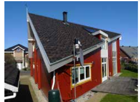
Heiko in the Netherlands installs a Vantage Pro2 on their environmentally friendly house.
